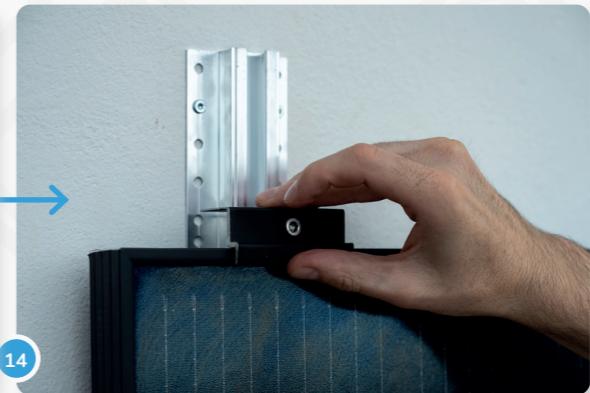
14 Schiene in Position bringen...
